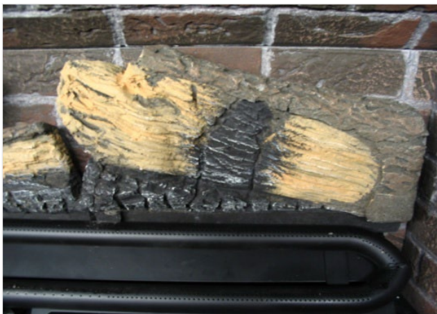
Log "B" installed correctly
